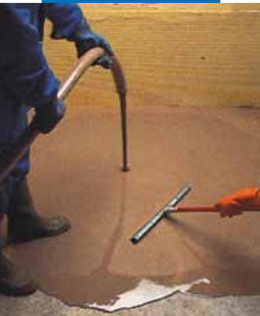
Application of Ultraplan with pump and squeegee
